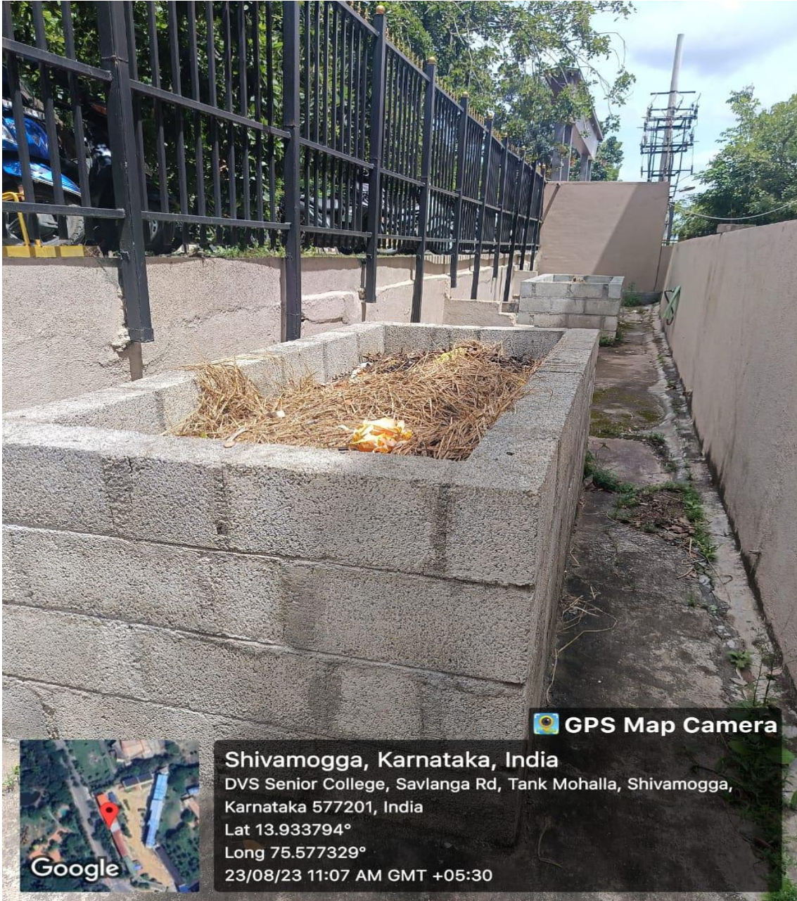
Bio degradable waste collected in fermentation tank
