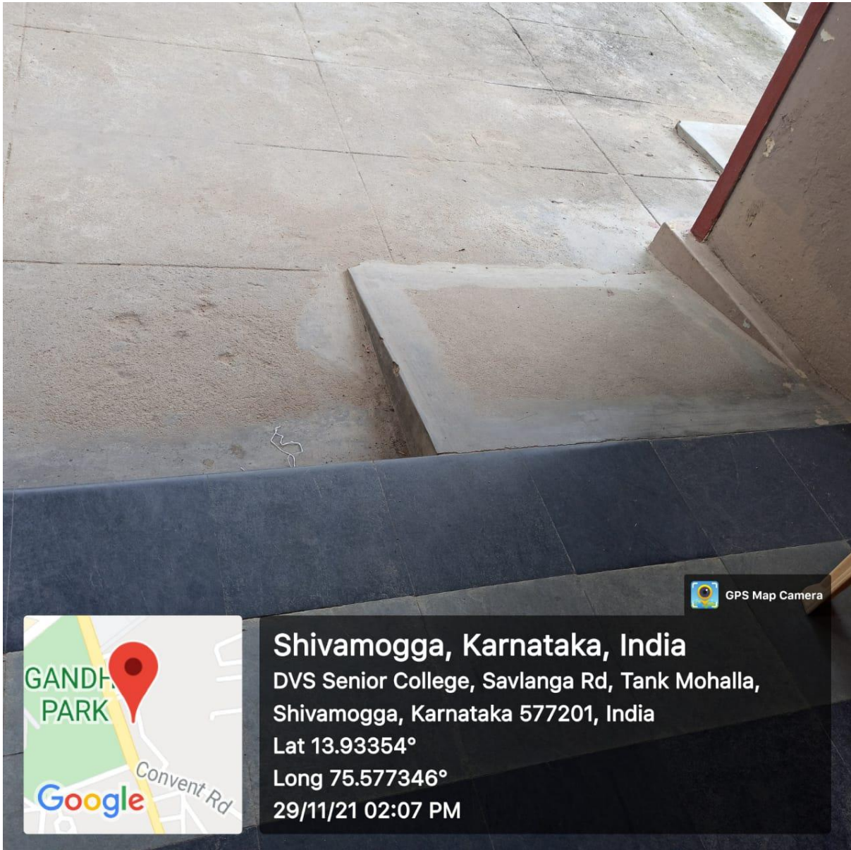
Ramp at the Entrance
