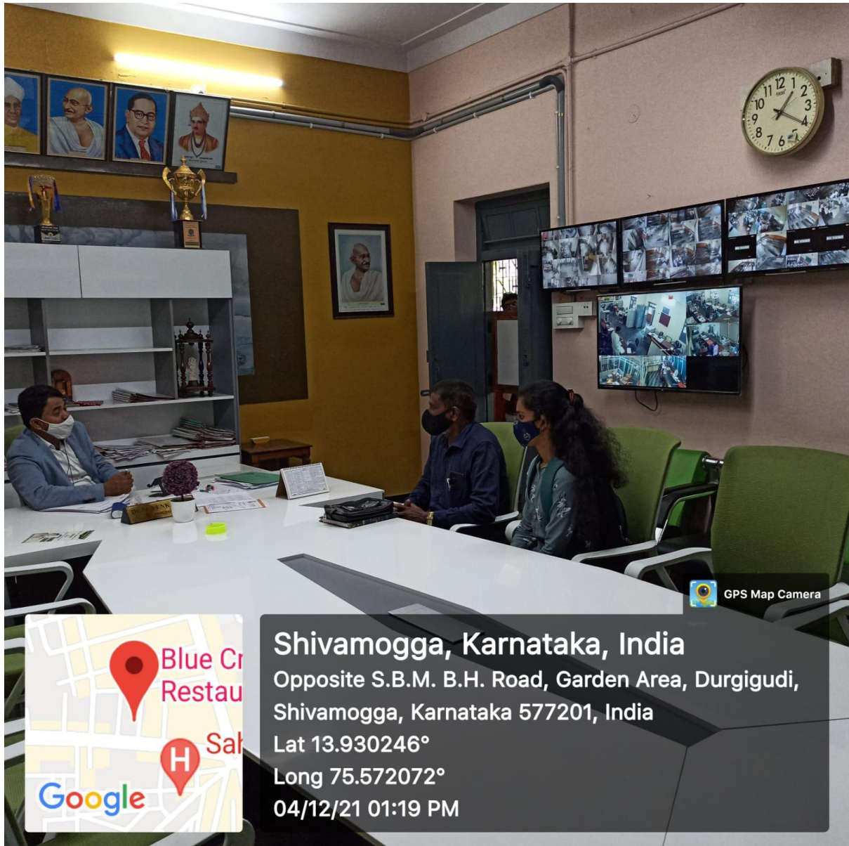
Display of CCTV Camera Footages in Principal Chamber for Monitoring
