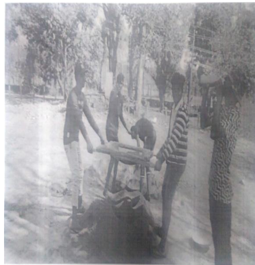
Rangamandira Construction Kamagari
