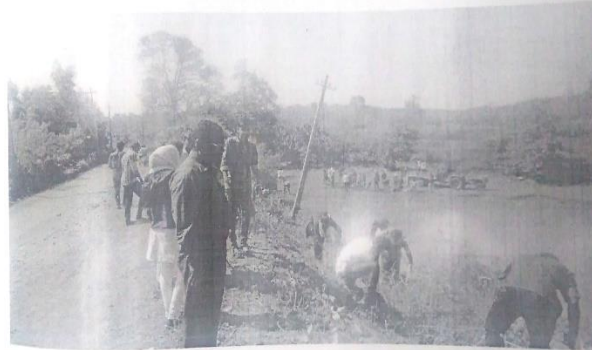
Cleaning of Tank Bunds of Tuppuru Grama
